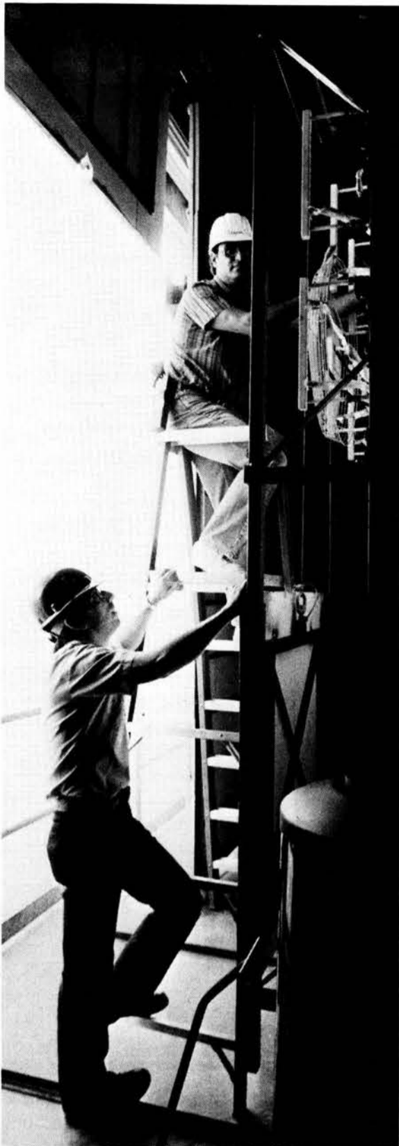
INSTALLING COMPONENTS on a test bed at the 220-ft. level at Sandia's Power Tower are Vince Dandini and John Aragon of Safety Systems Assessment Division 6445. The components, safety equipment used in nuclear reactor power plants, are being subjected to thermal fluxes up to 160 suns. The tests, part of the Hydrogen Burn Survival Program, are being conducted for NRC.
